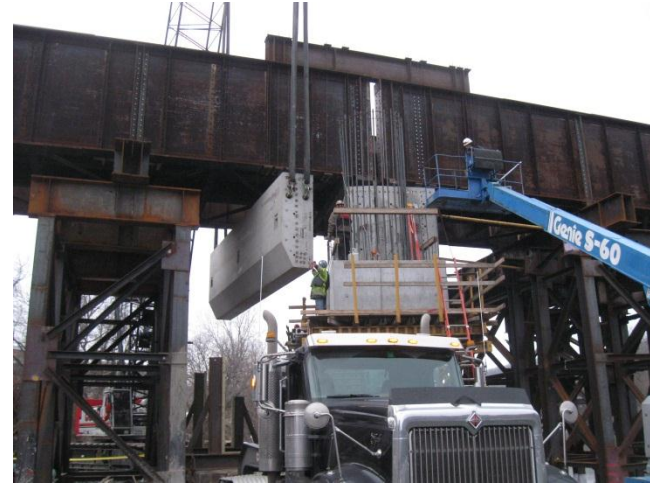
Precast Sandwich Beam Pier Cap (40 ton) – many details to coordinate
