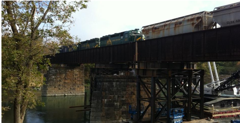
Hinged Cantilever Trains Running 42 Days After Response
