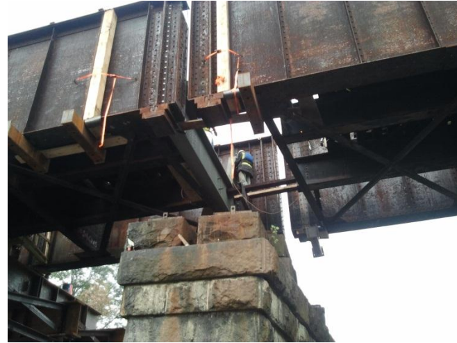
New Floor Beams – Easy Design, Tight Fab. Schedule (9/17-9/26) Required Increased coordination
