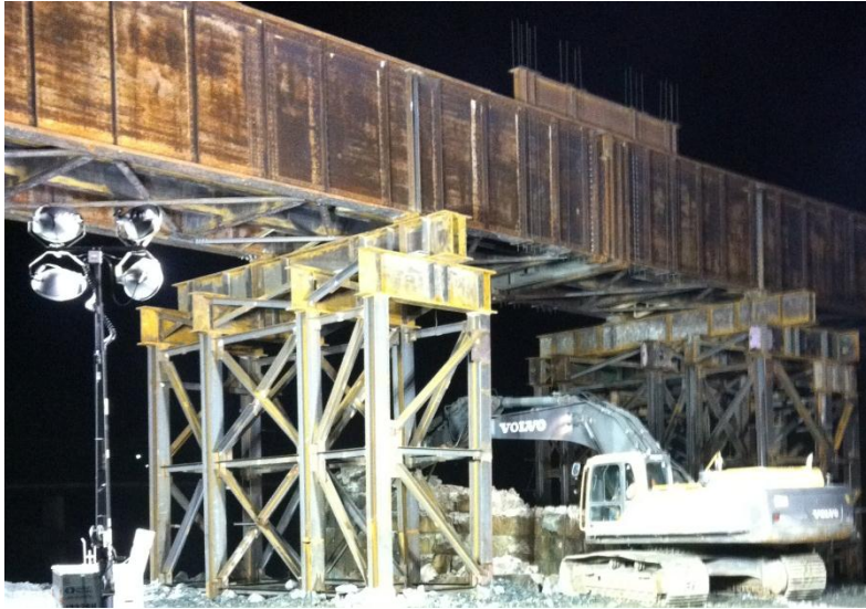
Shored Bridge to Cantilever Over Damaged Pier
