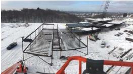
CCS is installing 400 tons of steel, bar joist and metal deck at this brand new 150, 000 sq. ft. elementary school.
